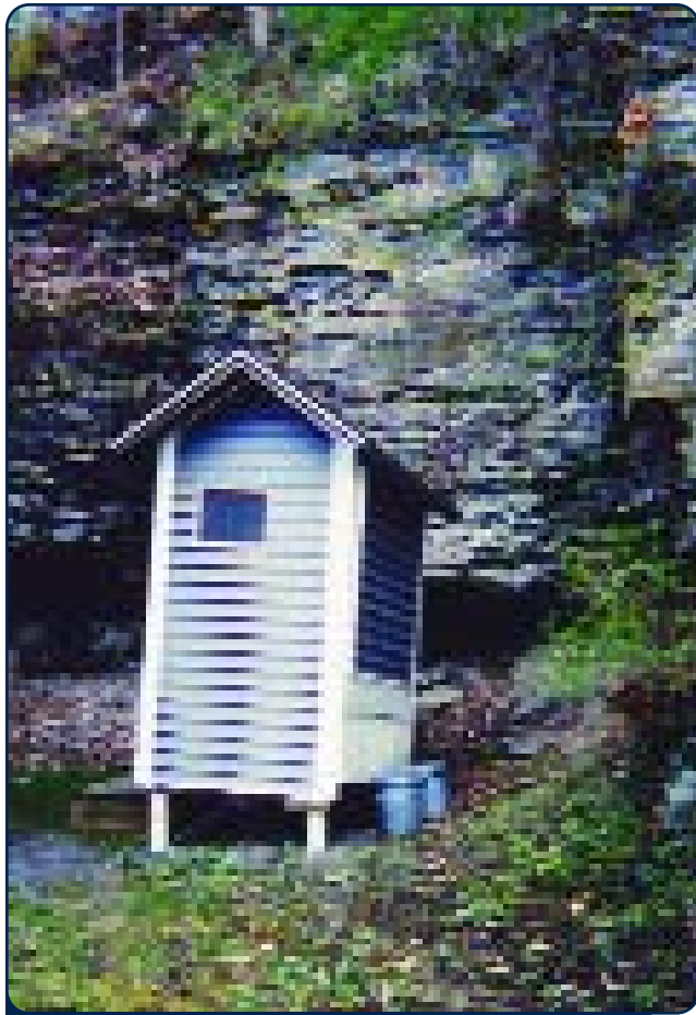
Privy behind a Skaneateles home shows the steep rocky terrain and limited land available for conventional onsite wastewater treatment systems. Photo by Patricia Miller.
